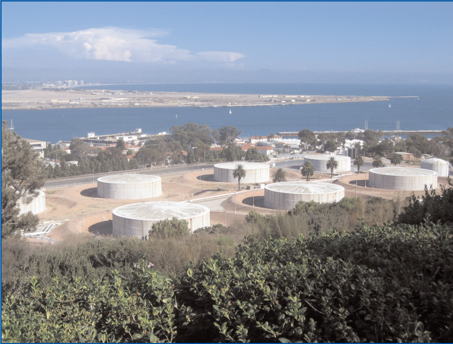
A view of the Navy's fuel tanks from the Trepte residence.
