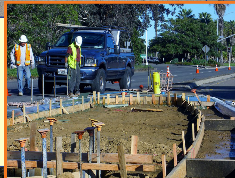
Framing for concrete edging.
