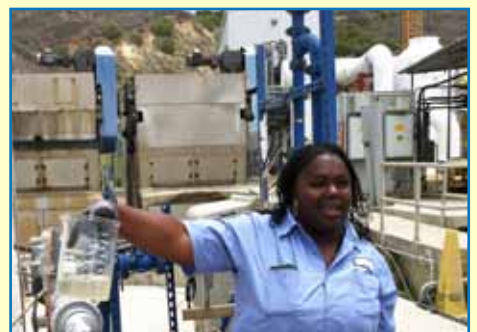
Childress and the "effluent." Note the clarity!
